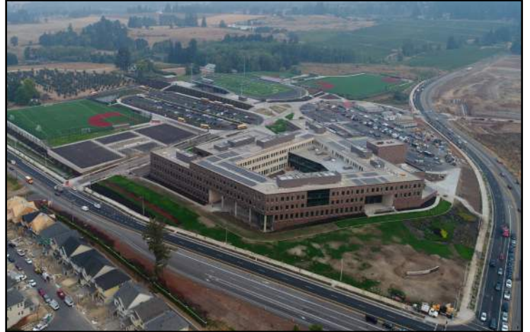
Aerial view looking northwest
