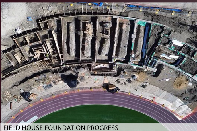
FIELD HOUSE FOUNDATION PROGRESS
