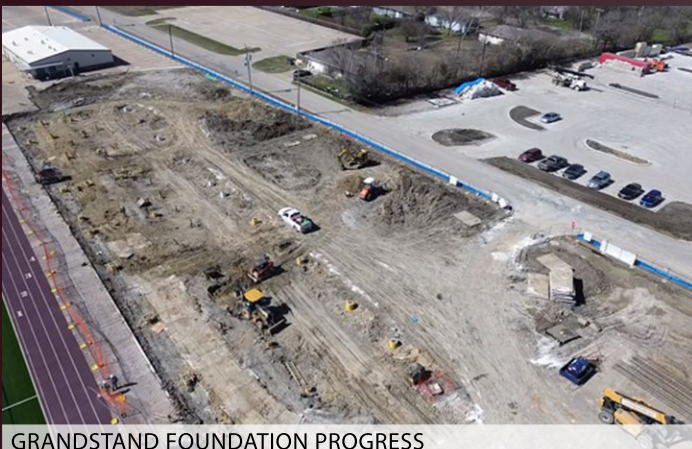
GRANDSTAND FOUNDATION PROGRESS
