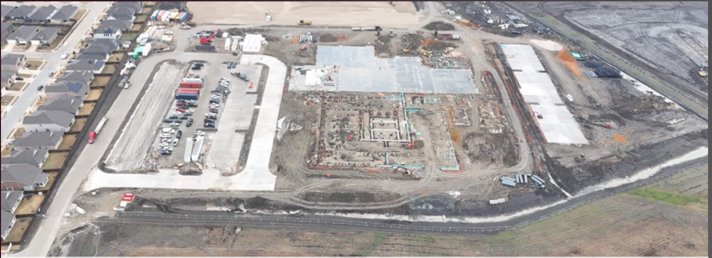
VIEW LOOKING EAST
