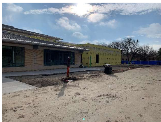
Sheathing Complete at Kitchen Addition at Alumni Hall
