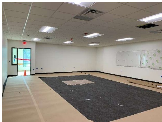
Carpet, Ceiling Tiles, and Markersboards Installed in Classroom at Heritage Hall
