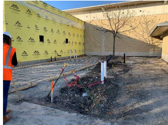
Prepping for Concrete Next to Kitchen Addition at Alumni Hall
