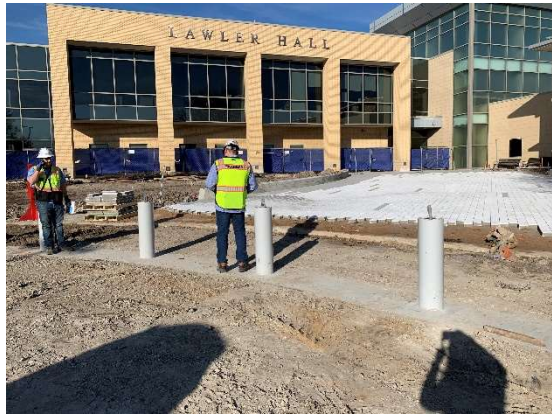
Pavers Installed at Lawler Hall
