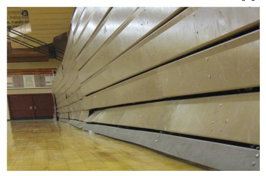
In addition, virtually all of the District's outdoor bleachers do not meet current safety and ADA standards; they need to be removed and replaced with new ones.
