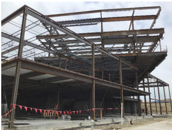
South View of North Building
