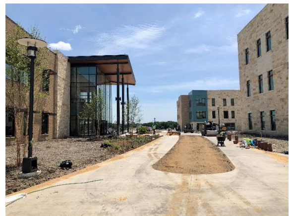
North View of Campus Quad Area
