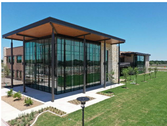
South View Aerial of Library Main Entrance
