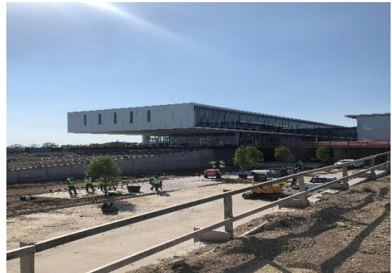
Trees Being Installed at South Garage Entry
