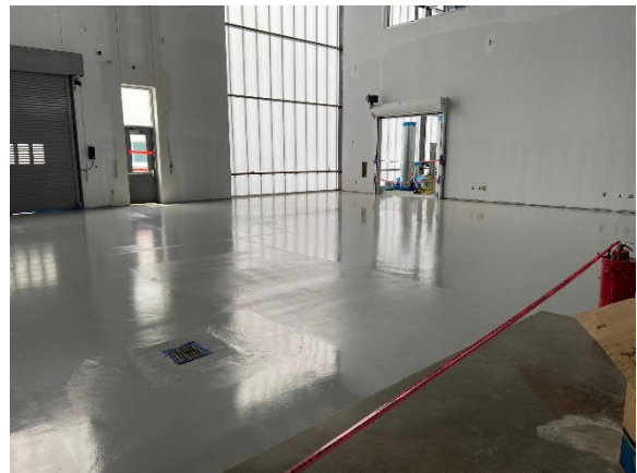
Epoxy Placed on Floors in Trade Bar D
