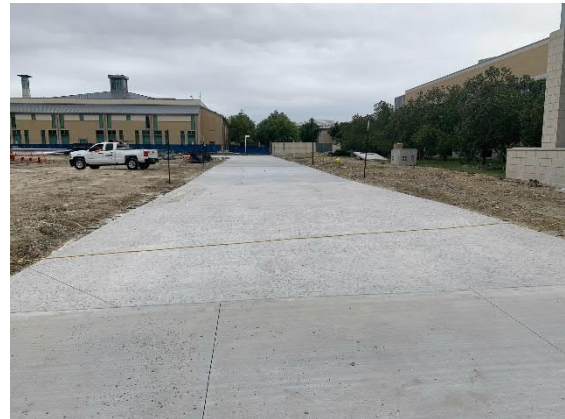
Firelane Poured in Quad Aea
