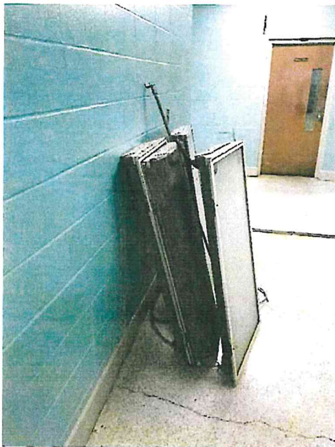
Remove demolished fixtures
