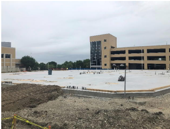
Concrete Poured in Area A
