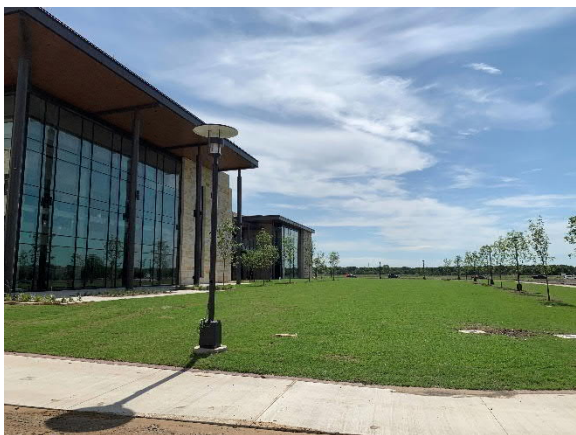
Sod Installed on South Side of Library
