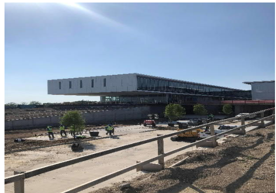
Trees Being Installed at South Garage Entry
