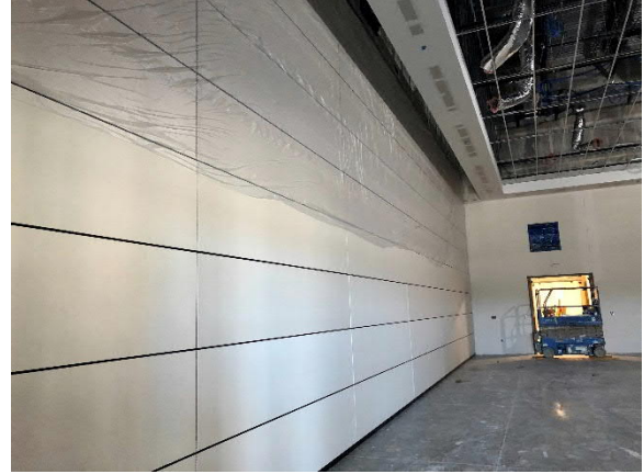
Partition Installed in Conference Center Room
