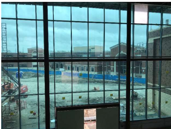
Window Installation in Welcome Center Atrium
