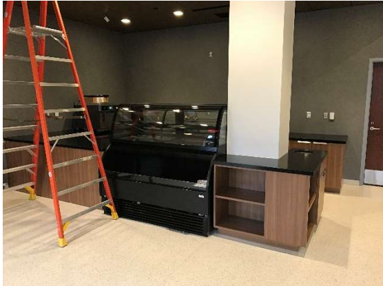
Starbucks Cafe Casework Installed
