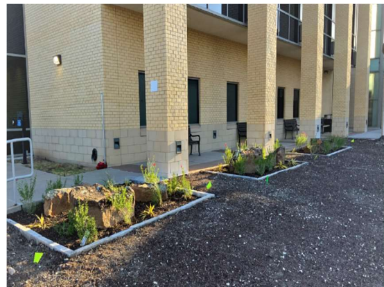
Landscape Planters Installed at Lawler Hall
