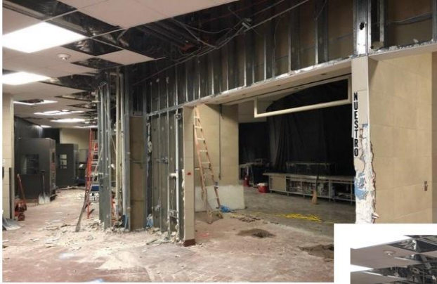
Braswell HS Kitchen Serving Line - Back
