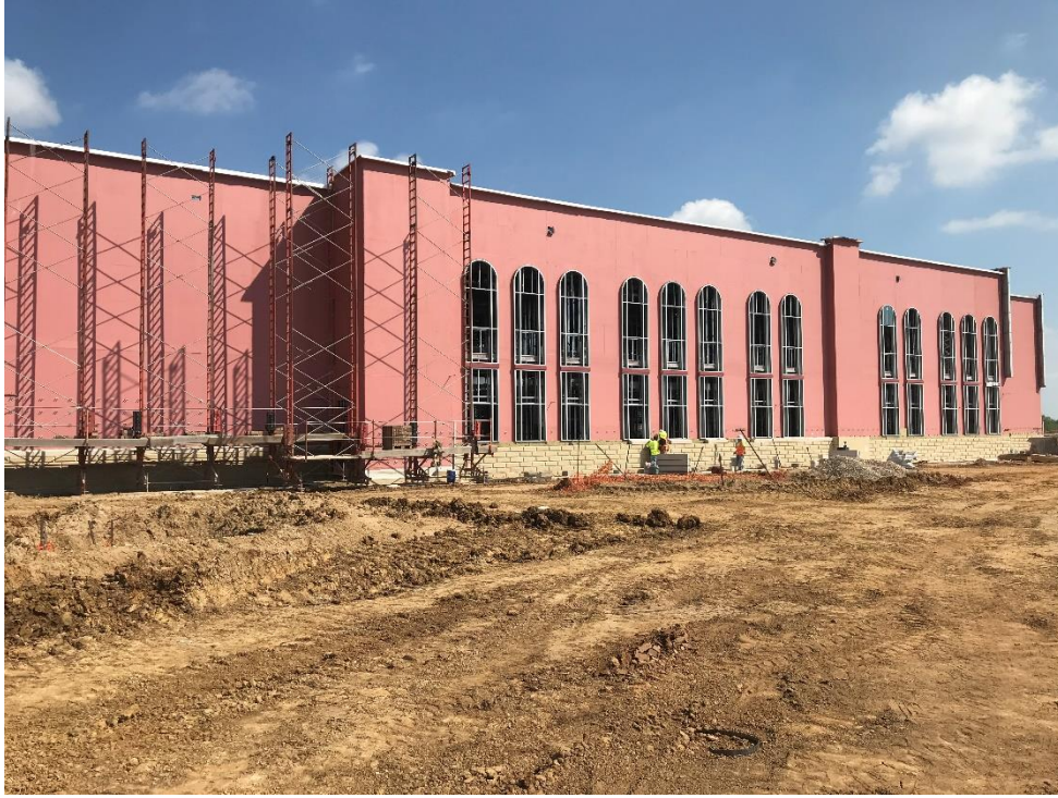
East Classroom Wing – South Exterior
