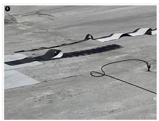
Seam repair strips are placed next to areas which have questionable adhesion.
