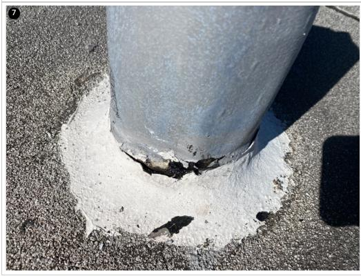
This is another soil stack with failed sealant.
