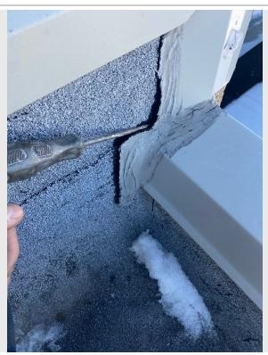
This corner flashing has a small opening which will be repaired.
