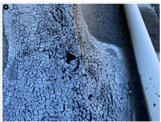
This corner seam has a small hole requiring repair.
