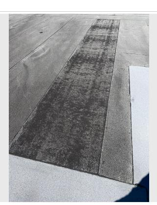
Small blisters and mineral granule loss are evident in this photo.
