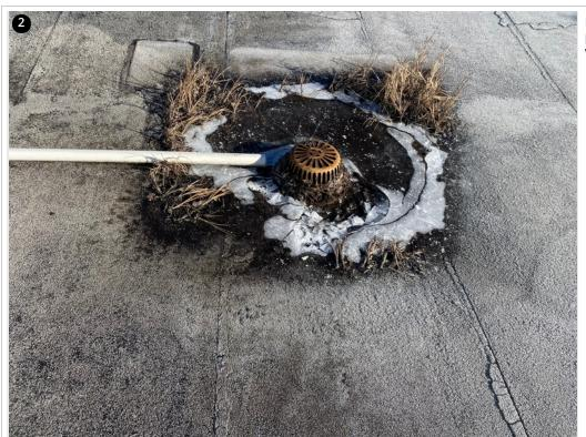
Debris is removed from drain sumps to prevent vegetation from penetrating the waterproofing membrane.
