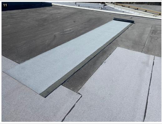
Repair material is relaxed prior to installation on the roof section.
