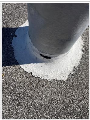
The sealant around this soil stack has failed and needs additional repair.
