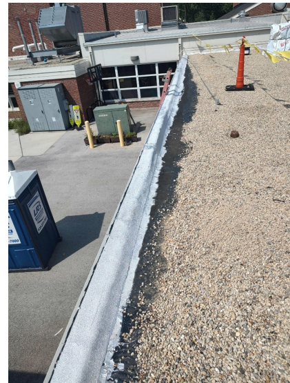
COPING REPLACED & NEW BALLAST IN PLACE
