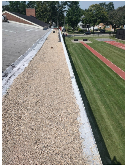
COPING REPLACED & NEW BALLAST IN PLACE
