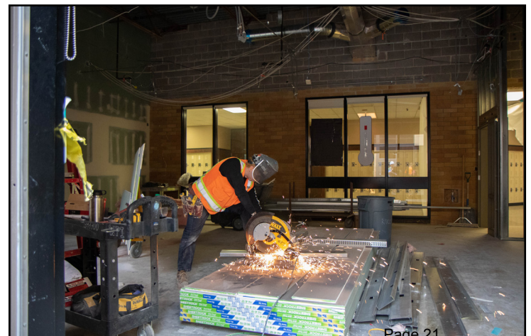
Lower classroom construction
