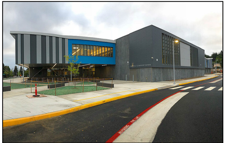
Front of building
