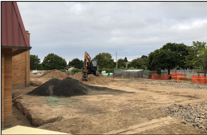
Concrete slab preparation where portables used to be
