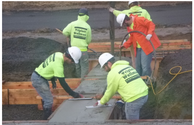
Pouring concrete footings
