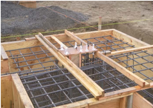
Rebar set for footings
