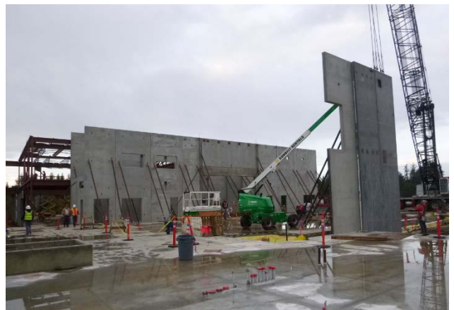
Precast panel installation
