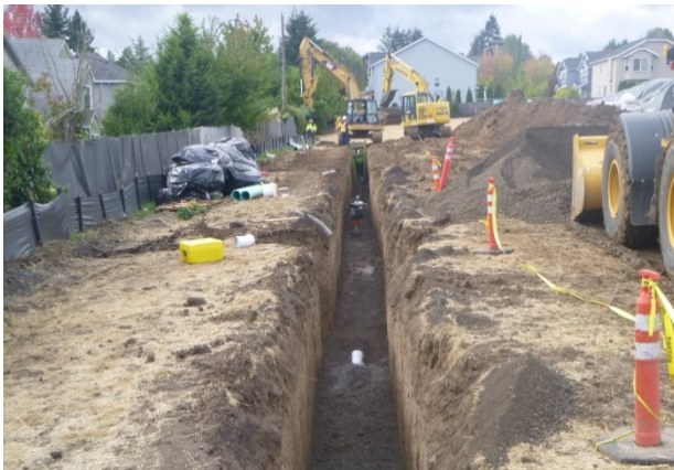
Stormwater pipe excavation
