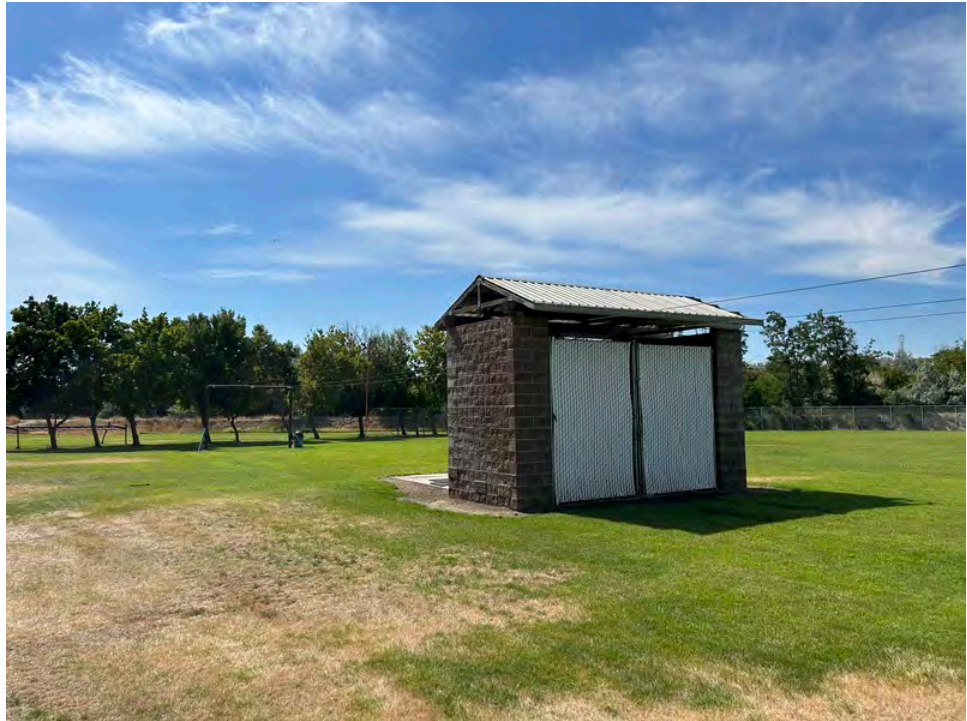
Photo 11. View of batting cage cover, located north of baseball field
