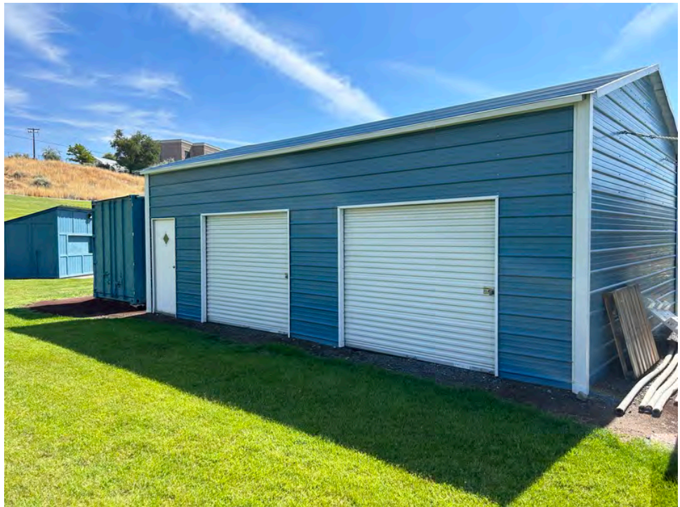
Photo 6. Equipment storage shed and shipping container, located west of baseball field
