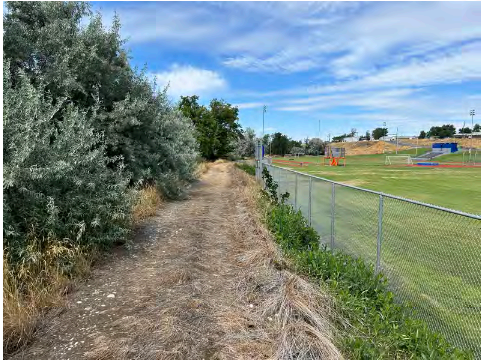
Photo 23. Stormwater berm extending along southern boundary, looking west
