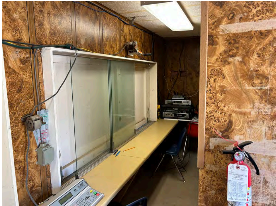
Photo 4. Interior of announcing booth
