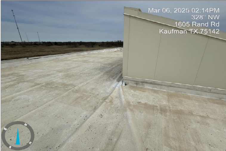
Fractured corners and seams.
