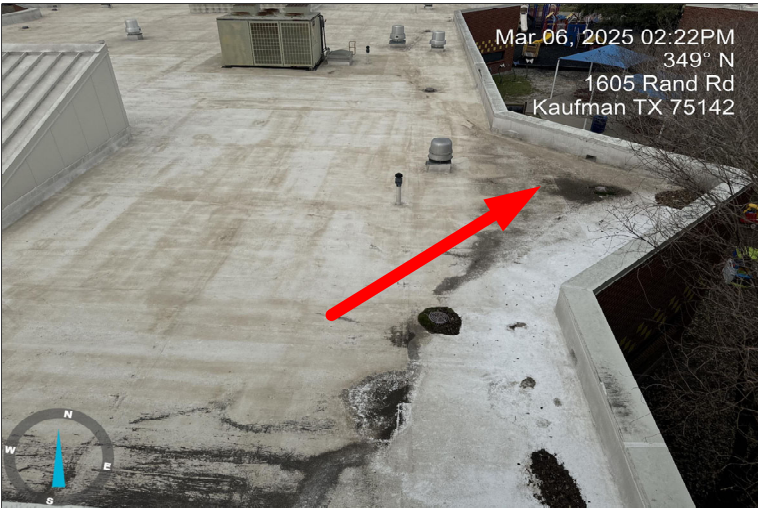
Severe ponding water around drains.
