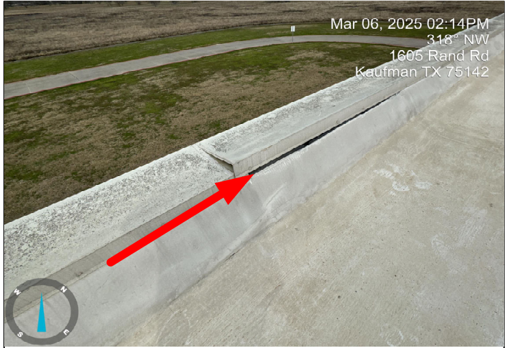
Fractured metal seams.
