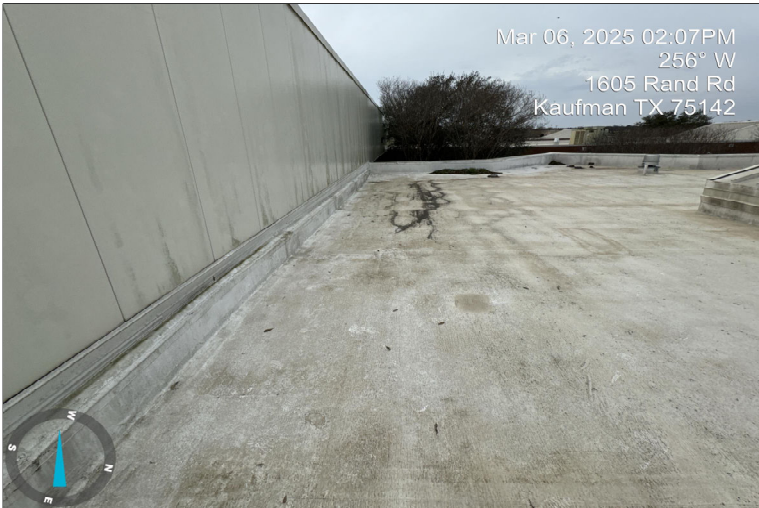
Membrane/Coating degradation.
