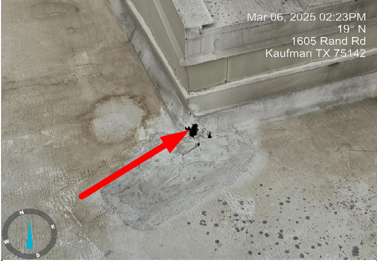
Severe corner flashing holes.
