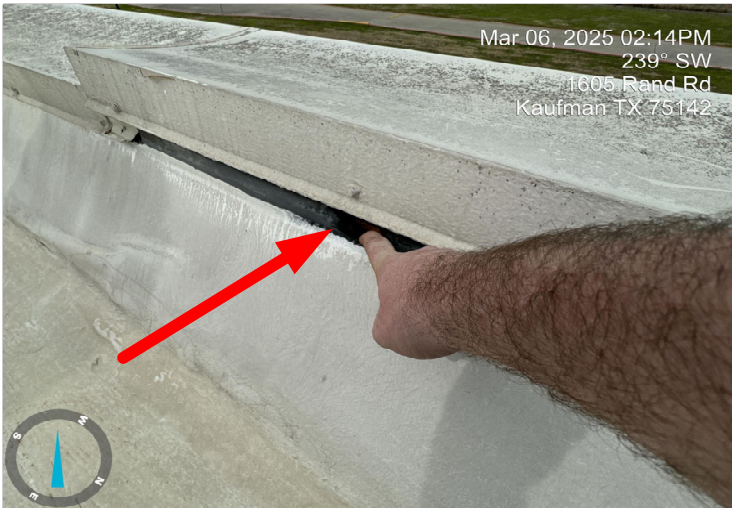
Complete seam shrinkage below coping.
