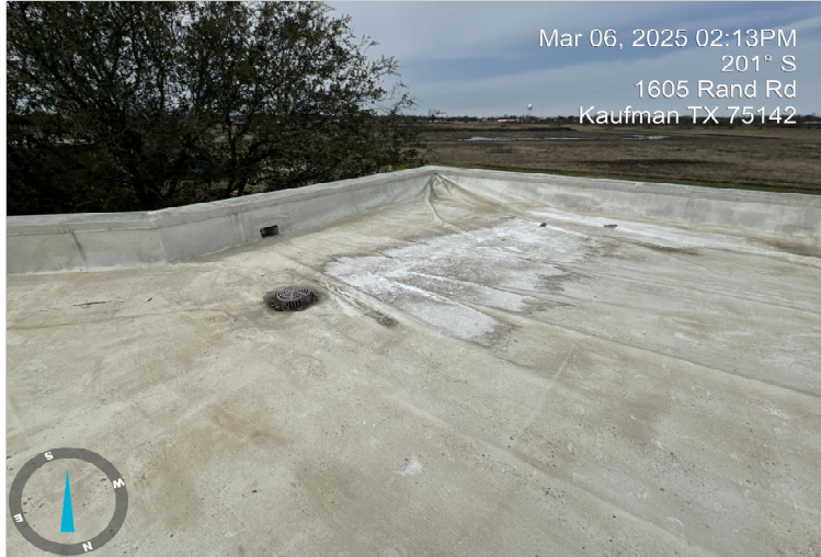
Single ply fully stretched from loading.
