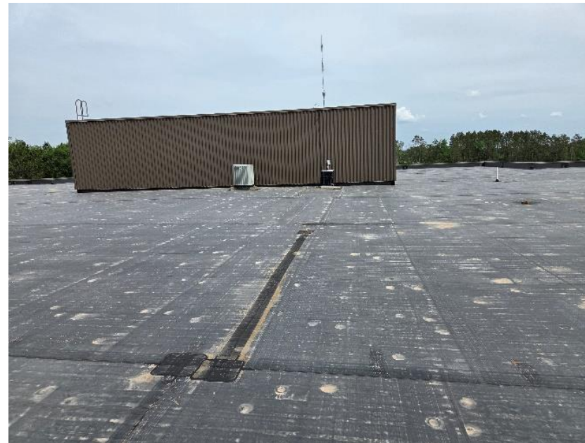
Fully adhered roofing.
