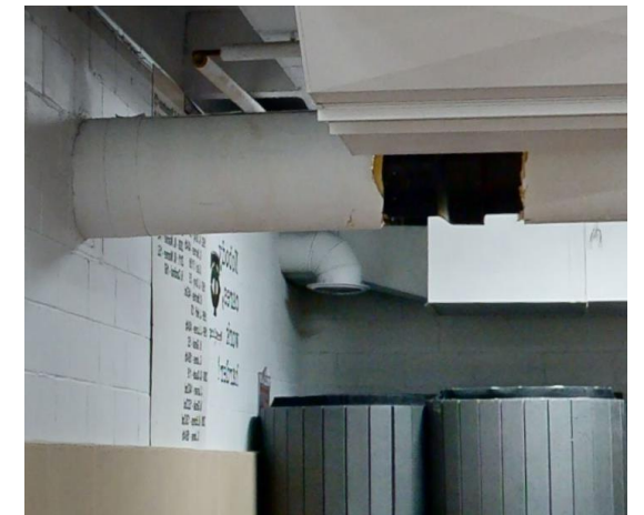
Small vent in the corner of the room.
