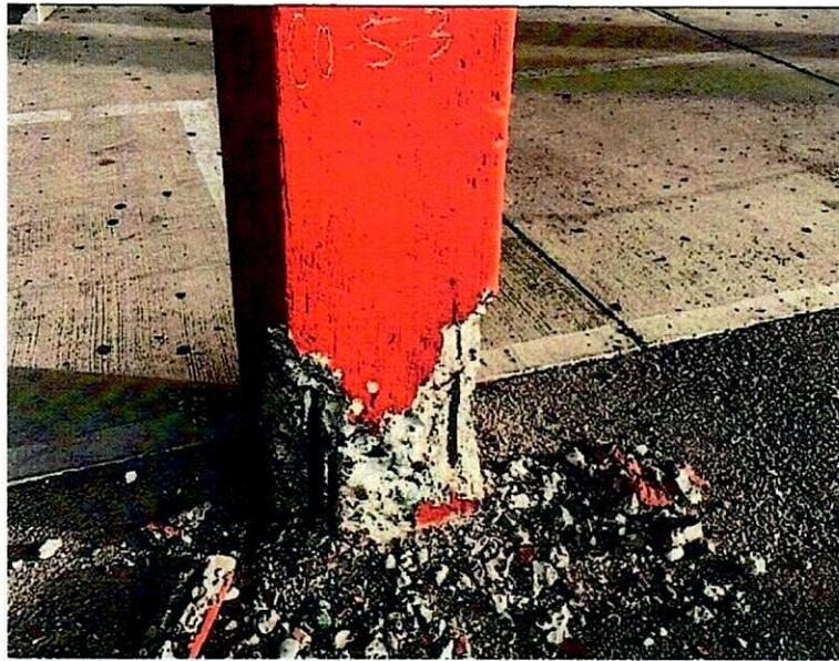
Photo #1: Column is Experiencing Spalled Concrete and Exposed Rebar.
