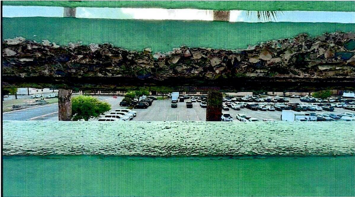
Photo 6: Zoomed In Photo of Louver on Press box Showing Exposed Rebar with Minor Oxidation.
