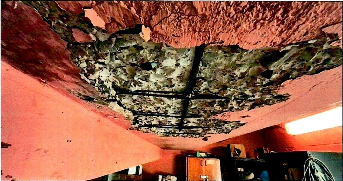
Photo 3: West Stands Bleacher Beam Underside Showing Exposed Rebar with Extensive Corrosion.
