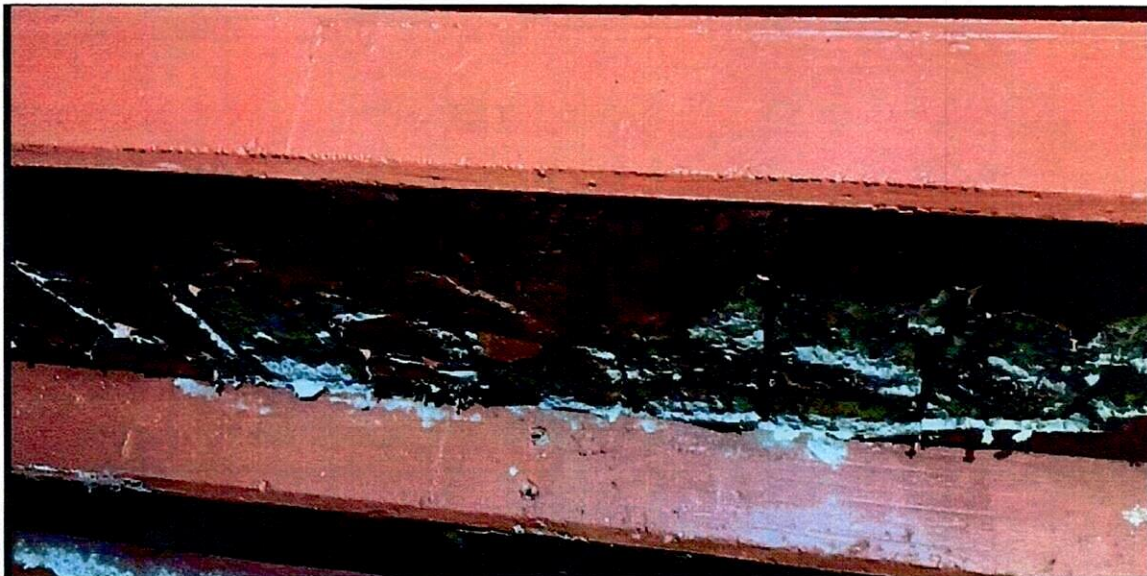
Photo 4: East Stands Bleacher Beam Underside Showing Delamination and Spall with Moderate Corrosion.
