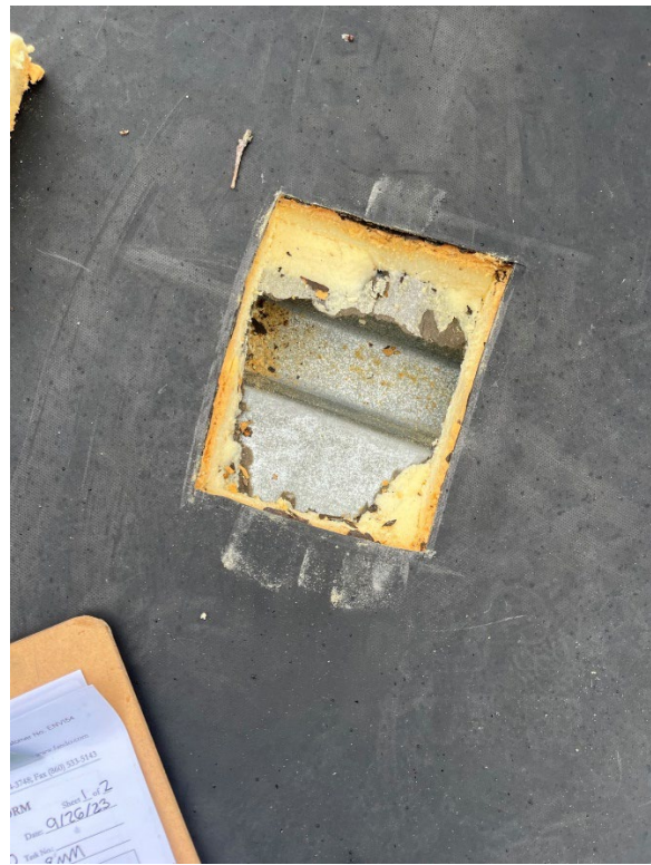
Roof K – Field
