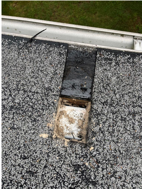
Roof D – Perimeter
