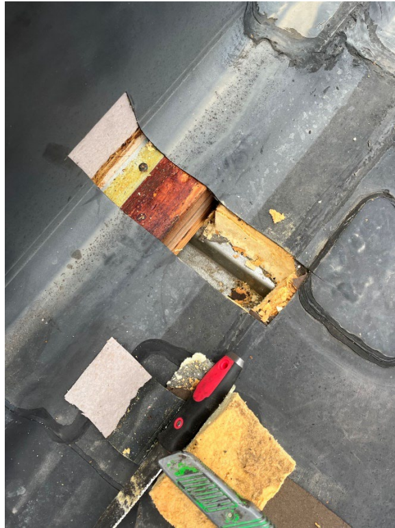
Roof K – Penetration
