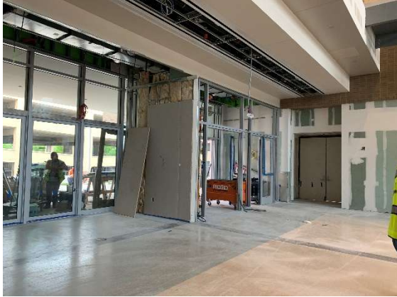
Main Entrance at North Side of Building
