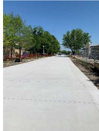
Fire Lane Poured, North to South View
