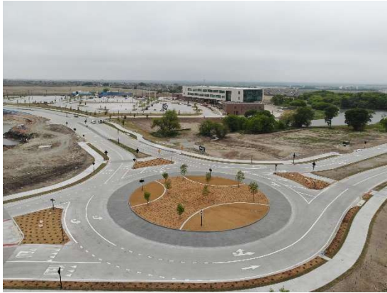
Roundabout at Choate Parkway/Kinship Parkway
