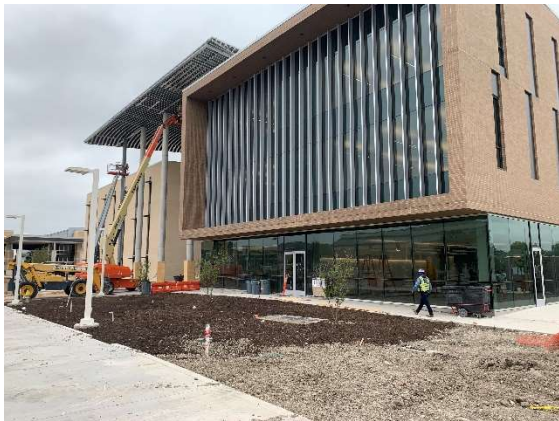
South Façade of Building
