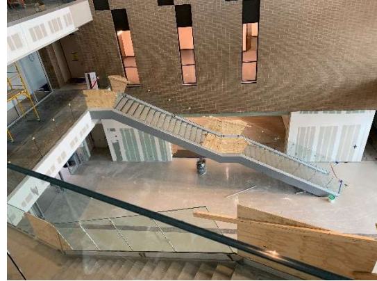
Glass Handrail Installation at Stars in Atrium
