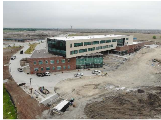
April Aerial Looking Northwest
