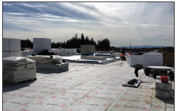
Roofing above Gym
