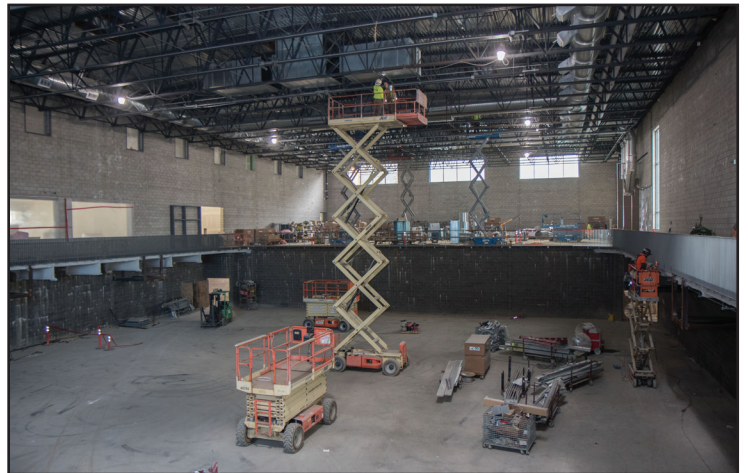
Main gym/Upper gym
