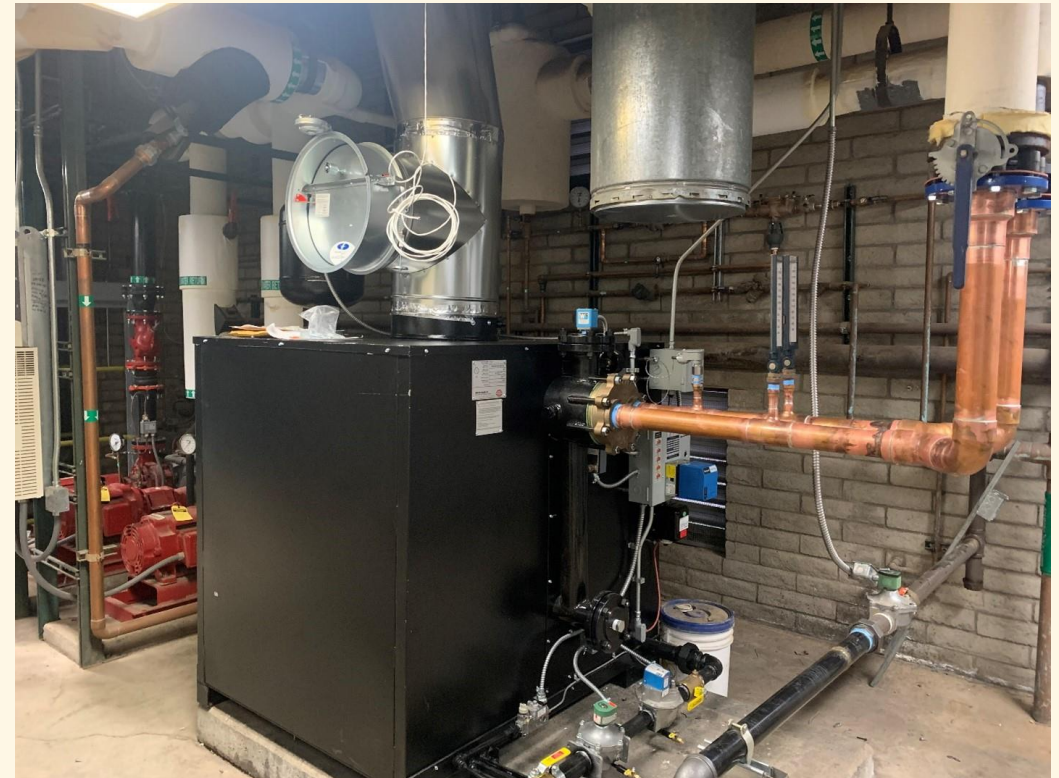
Coronado K-8 Boiler Replacement
