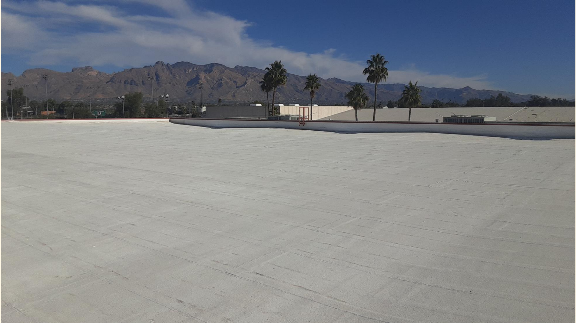
AHS – Main Gym Roof Replacement
