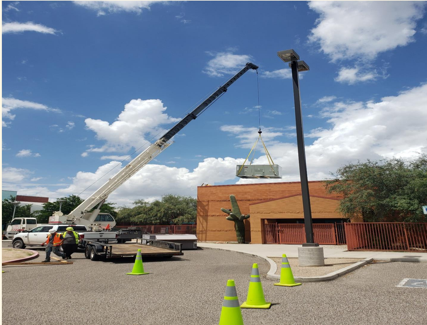
Prince ES Mustang Room HVAC Replacement
