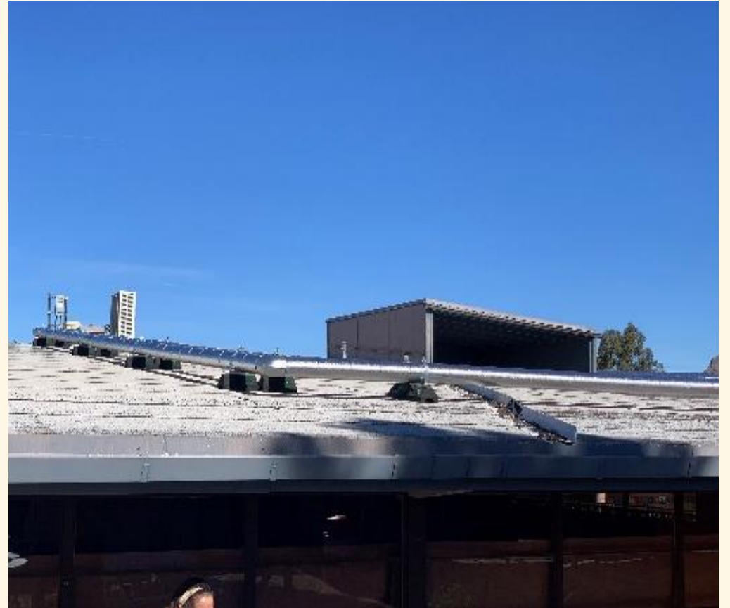
Harelson ES Hot Water Line Replacement
