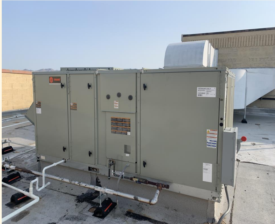
Copper Creek ES Kitchen HVAC Replacement
