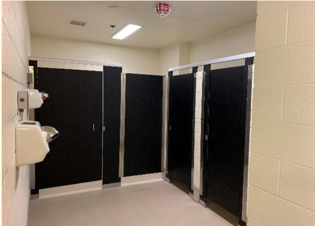
AHS Locker Room Improvements
