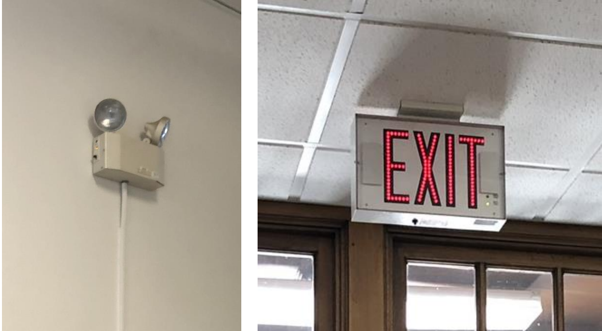
EXISTING EGRESS LIGHT FIXTURE AND EXIT SIGN.
