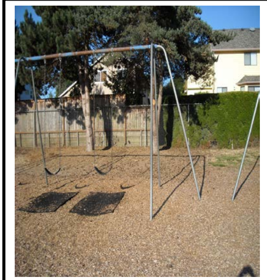
Old Swing Set with Evidence of Rusting
