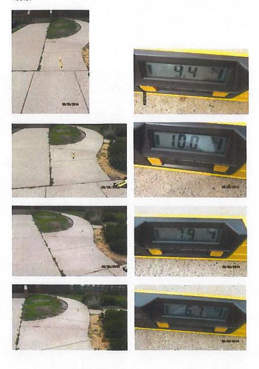
10. There is a change in level at the base of the ramp, where the accessible route meets the ramp that exceeds ½ inch [1" gap]. IAC § 400.310(a); Standards § 206.1.
