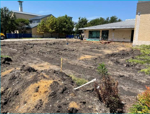
Grading of Foundation for Kitchen Addition at Alumni Hall
