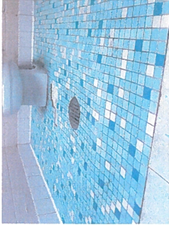
Classroom Student Restroom
