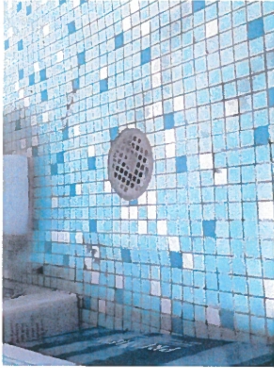
Classroom Student Restroom
