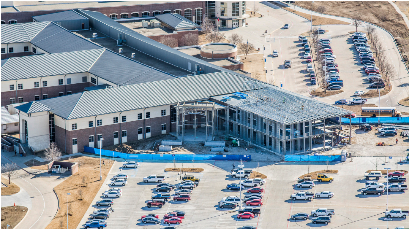
Area C - Framing
