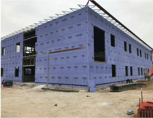
Area C - Exterior Sheathing
