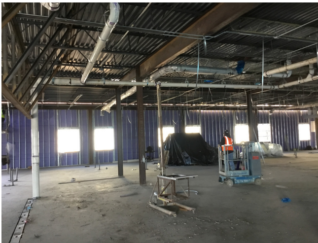
Ninth Grade 2nd Floor plumbing and Overhead rough-ins
