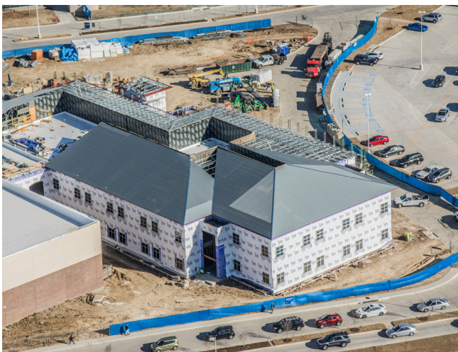
Northwest view of Area D & E rooftop
