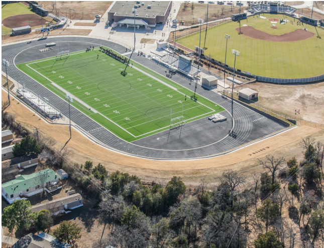
Track Striping Completed
