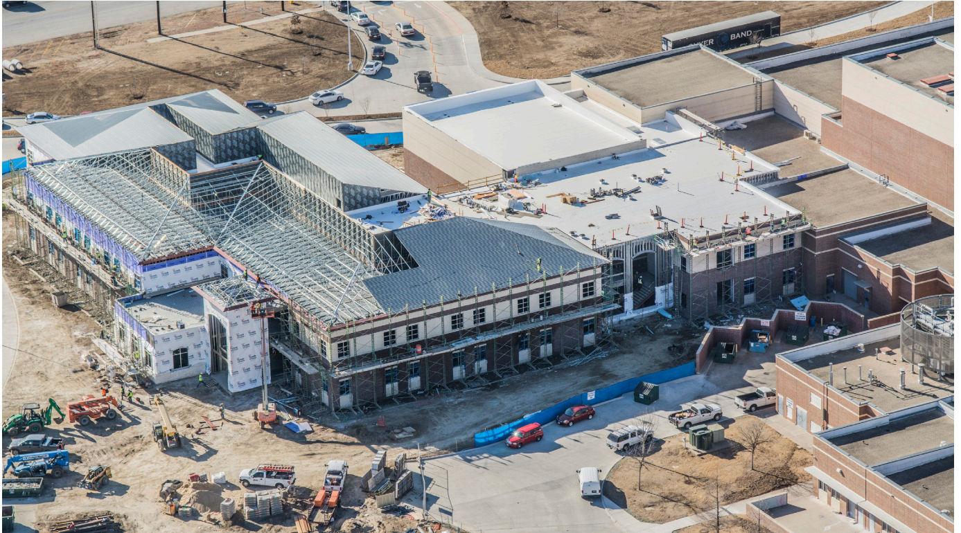
Southeast view of Area D & E masonry and rooftop
