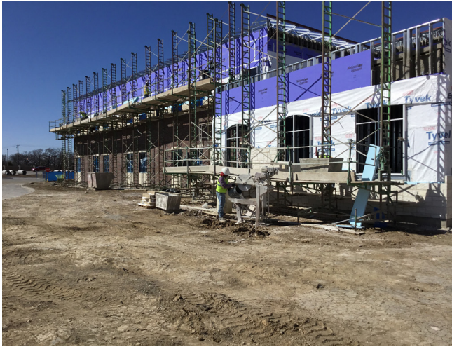
Exterior Masonry in progress
