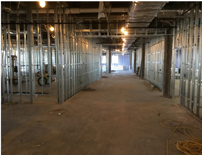
Interior Framing and Overhead Utilities
