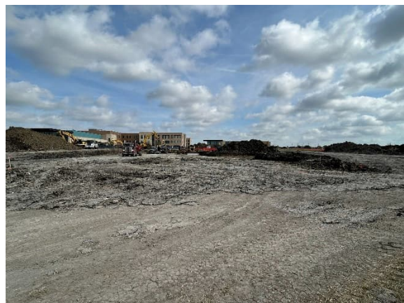
Site Excavation and Grading
