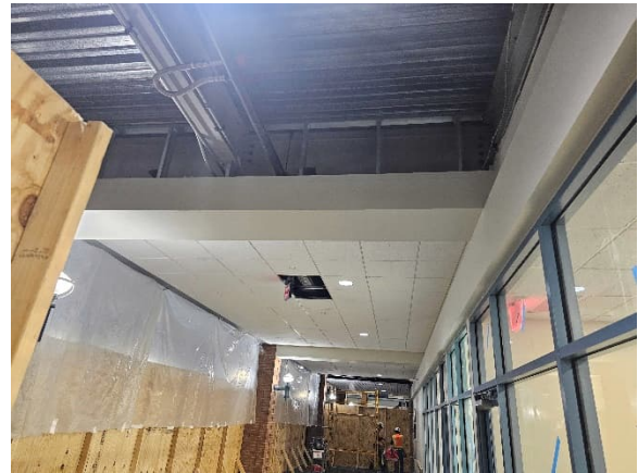
Ceiling Outside Welcome Center
