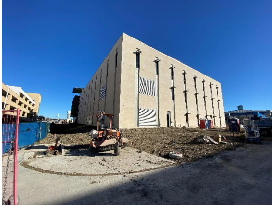
NW View of Building
