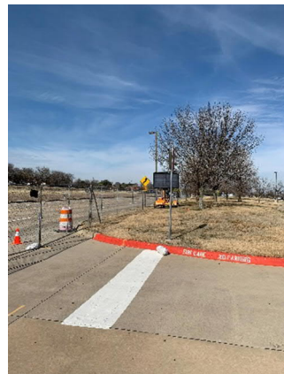
West View of Fencing Installed Along Community Ave
