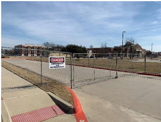
NW View of Fencing Installed for Construction
