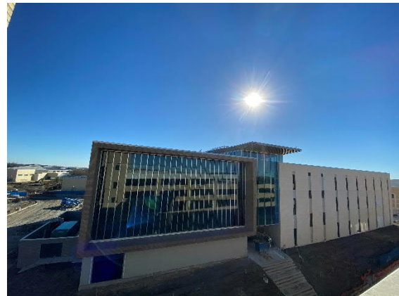
North Curtain Wall
