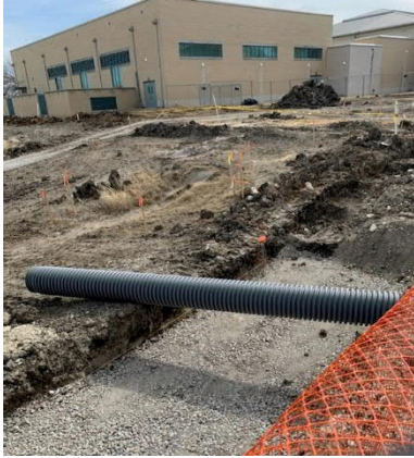
8" Storm Pipe for Retaining Wall, North of Alumni Hall
