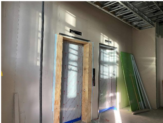
Elevators Installed at SE End of Building
