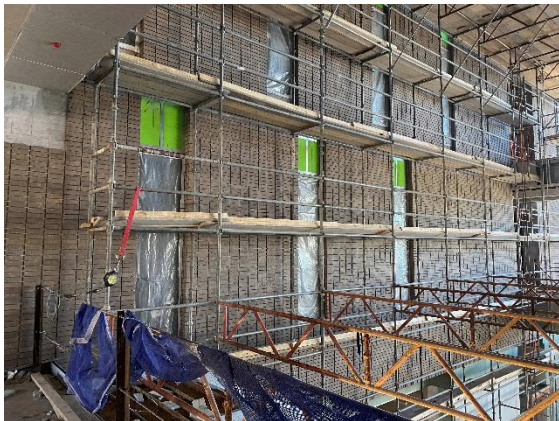
Thin Brick Installed at East Atrium Wall
