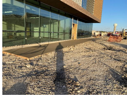
Sidewalk at SE Corner of Building
