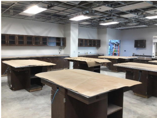
Science Lab Casework Installed
