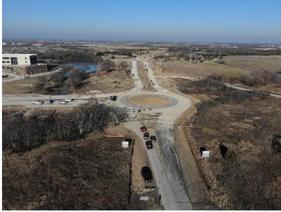
Roadway at West Entrance of Campus
