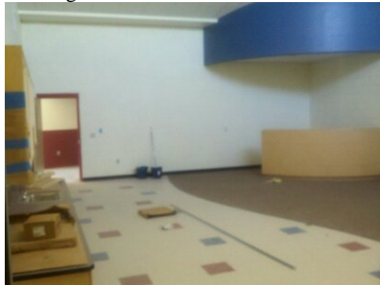
New Rillito Classroom
