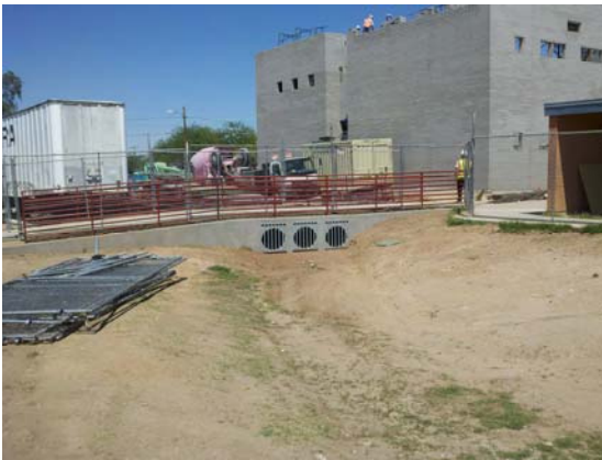
New ADA Walkways to Playground
