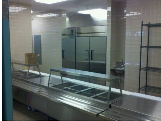
New Kitchen Serving Line
