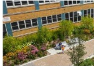
Asphalt Removal & Landscaping
