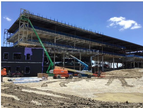
South View of North Building
