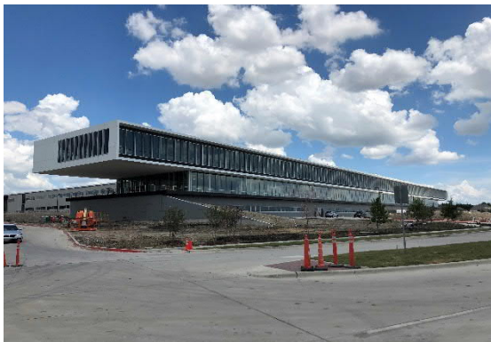
NW View of Academic Building from Bending Branch Way
