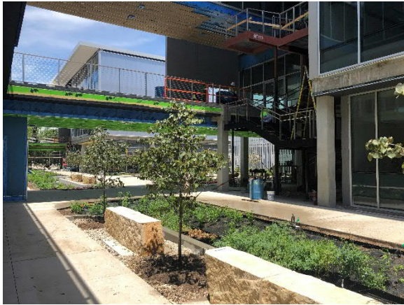
Bioswell and Building C Bridges
