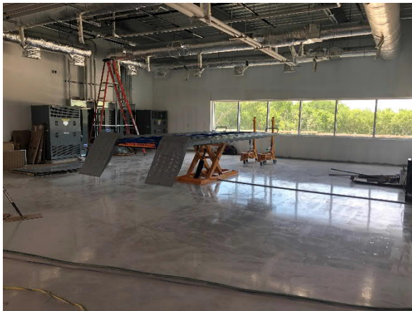
Trade Bar D Car-O-Liner Lift Installed
