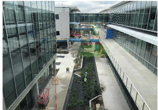
South View of Bioswales and Bridges
