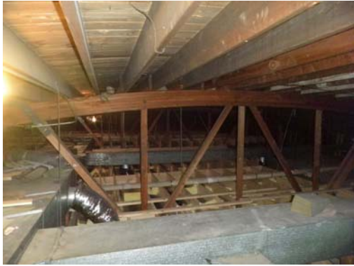
Bowstring Trusses at South West Area
