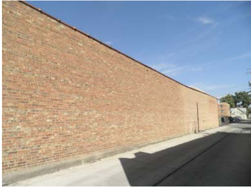
East Masonry Wall is in Good Condition
