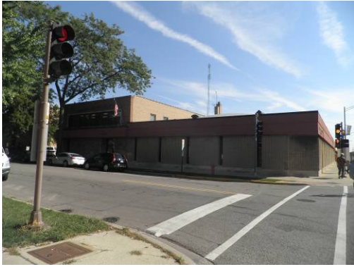
Exterior Split Face Masonry
