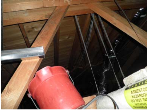
Bowstring Trusses Above Second Floor
