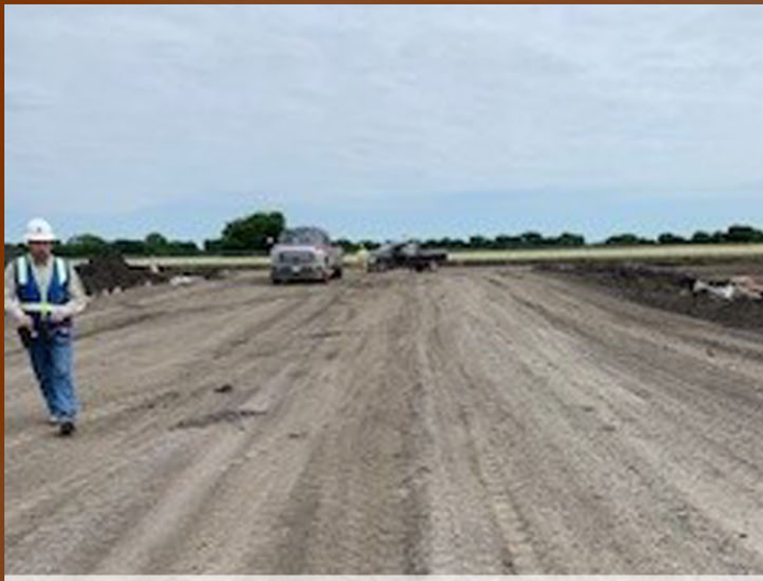
PAVING - ROUGH GRADING AT FIRE LANES/DRIVES
