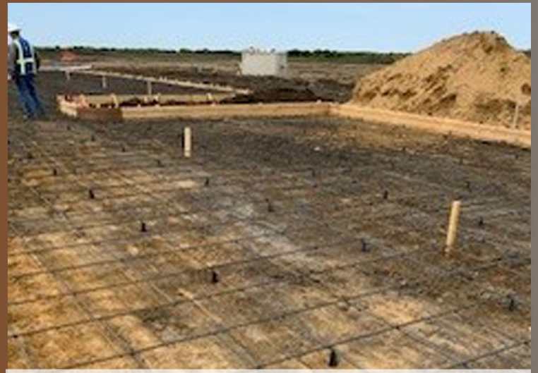
PAVING - REINFORCING AT PARKING LOT AREA
