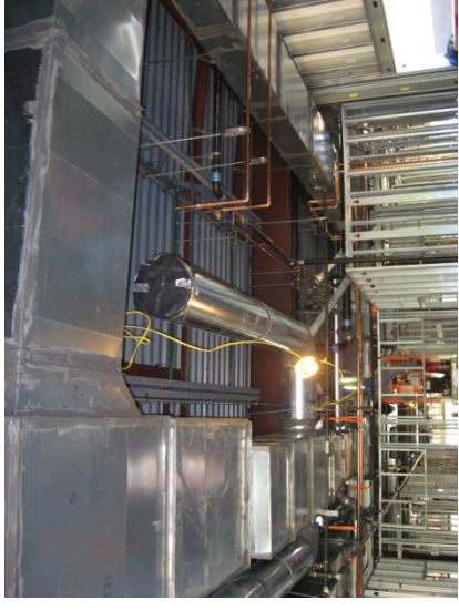
Mechanical ductwork installation
