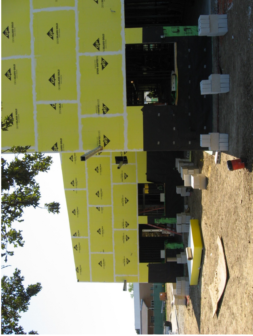
Preparation to begin masonry installation
