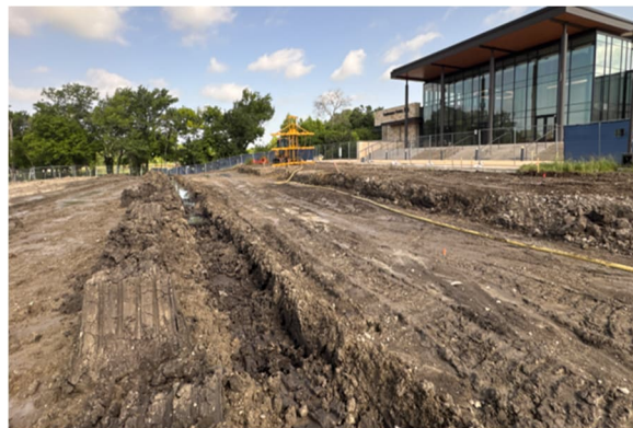
Grading for New Plaza
