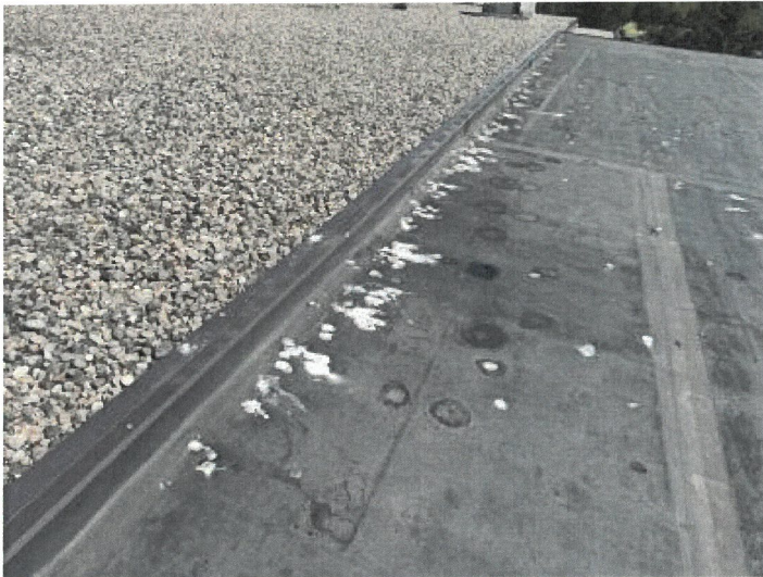
Bird Droppings-Contaminating Roof area
