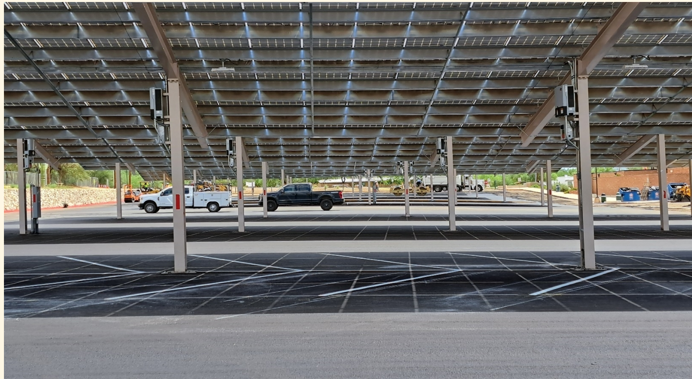
CDO Parking Lot Reconstruction
