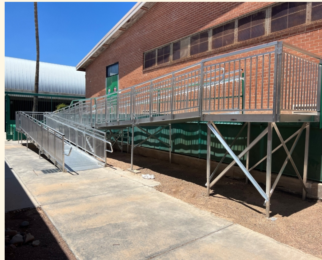
AHS D Building Access Ramp
