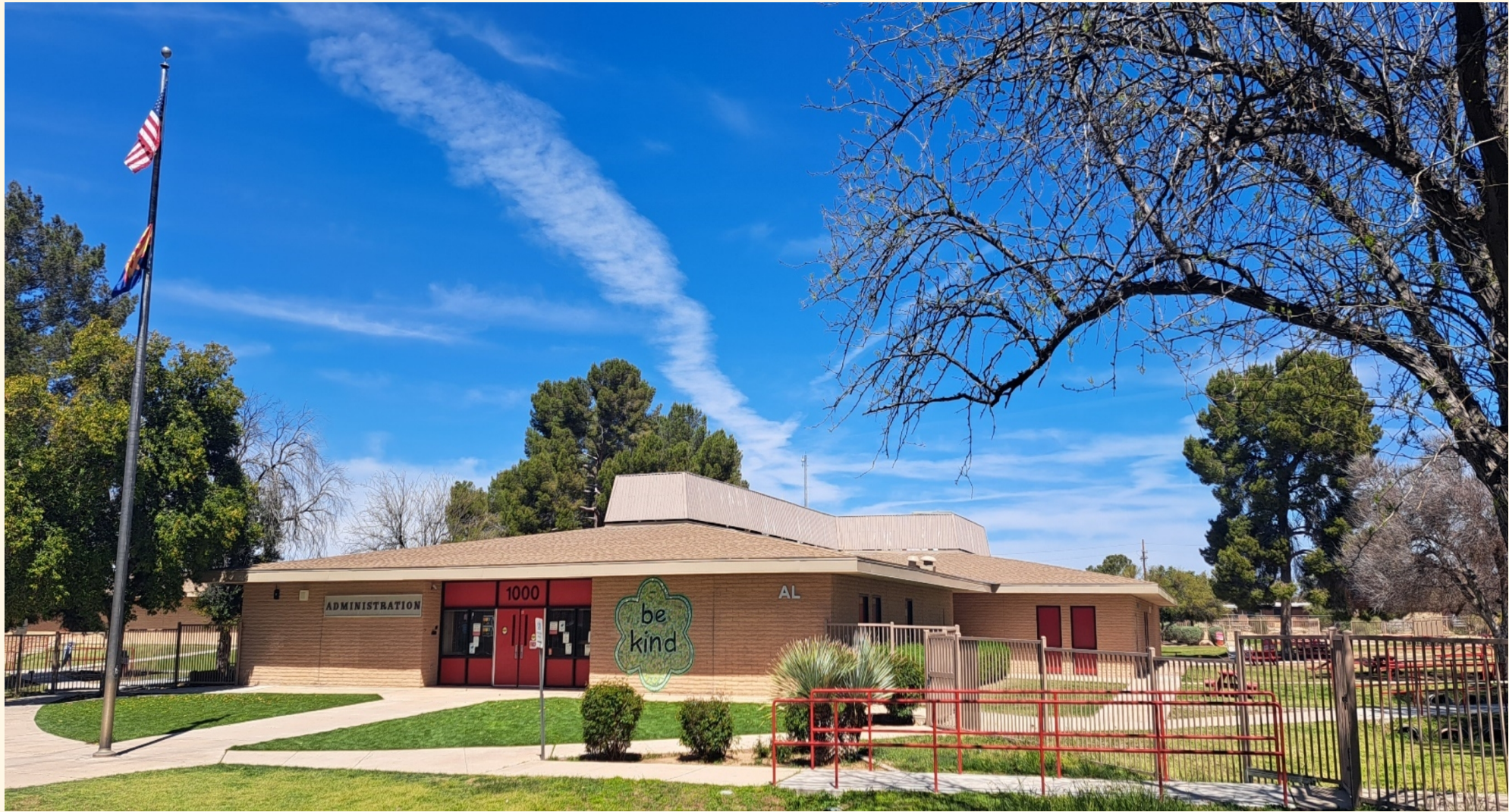
Cross Campus Roof Replacement
