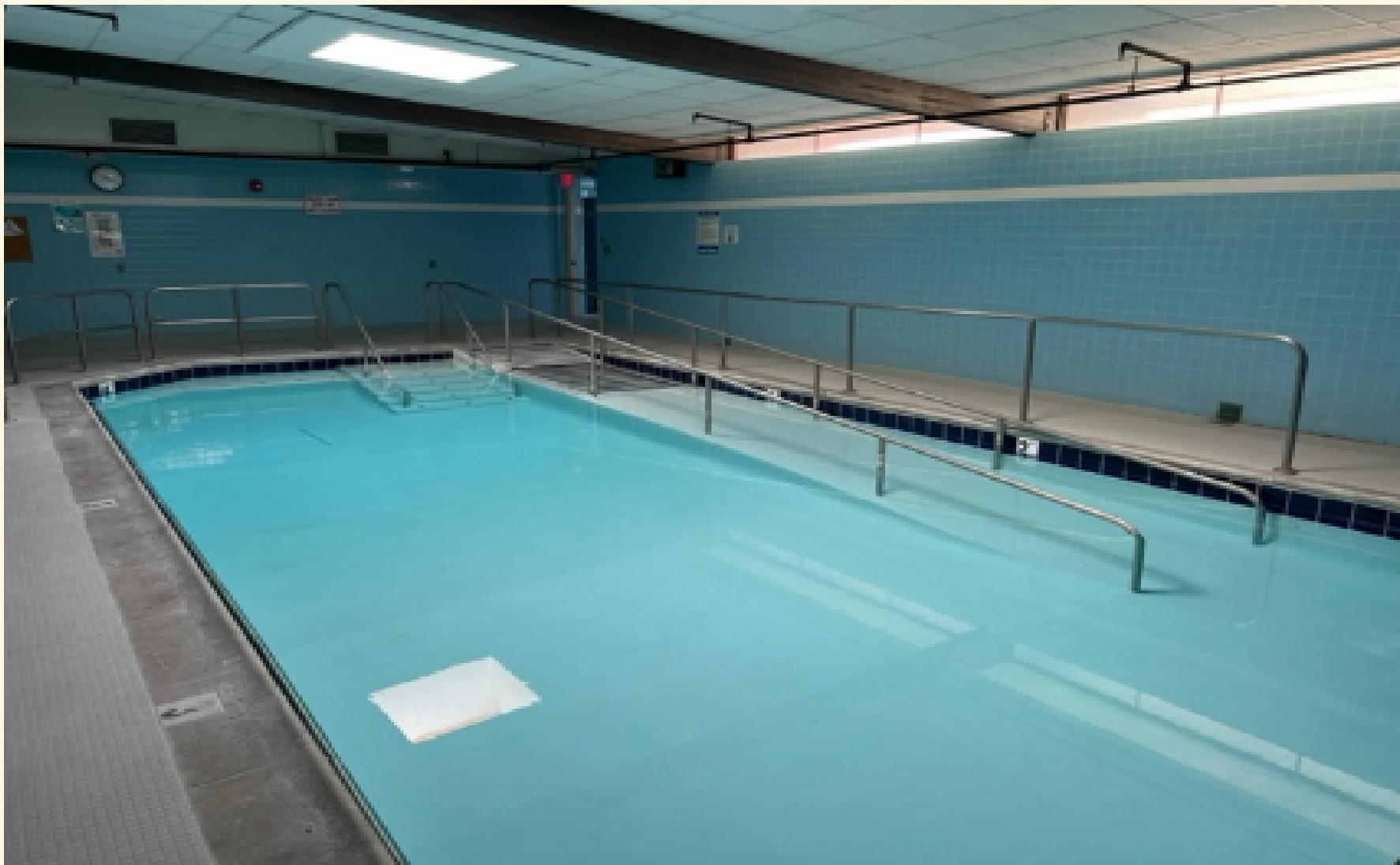
Rillito Pool Re-Plaster
