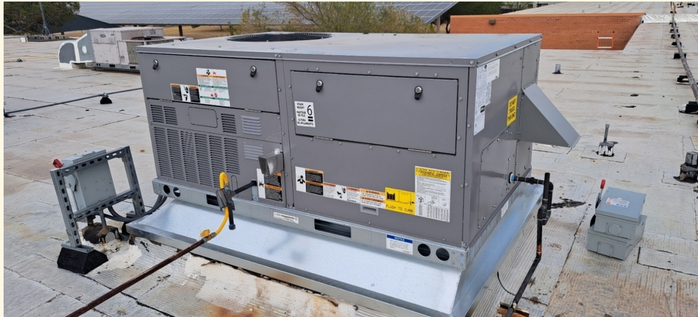
Prince Classroom 19 HVAC Replacement
