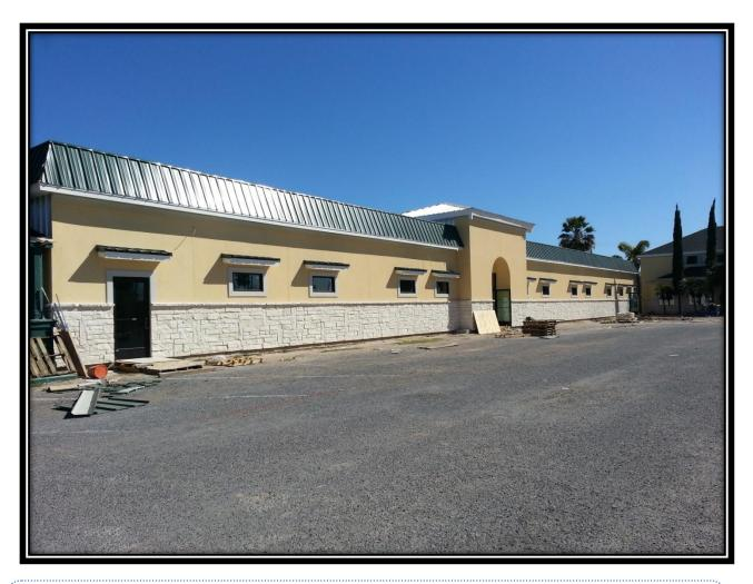
Pictured is the exterior of the building completed with stucco and stone. The small windows face the cubicle areas.
