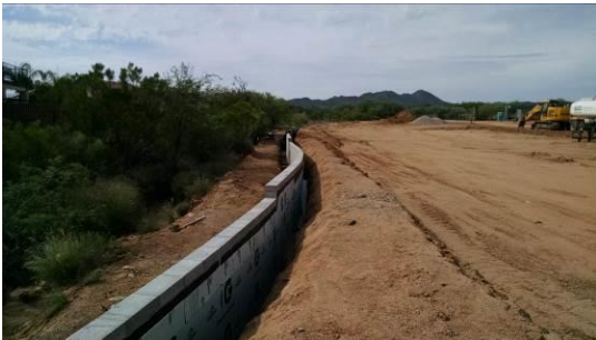
West side retaining wall complete
