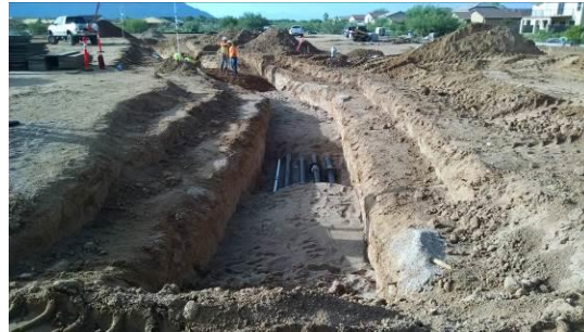
Chiller pipe trenches being backfilled
