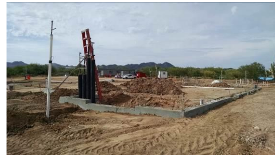
Footings and stem walls at 100 building
