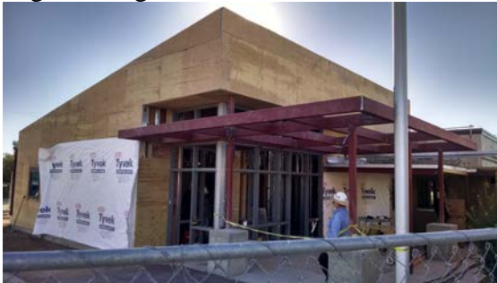
HR Dry-In and Interior MPE Rough-In
