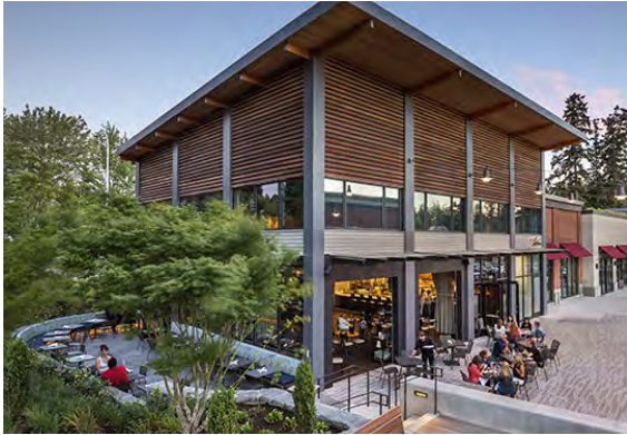
Examples of new commercial buildings
