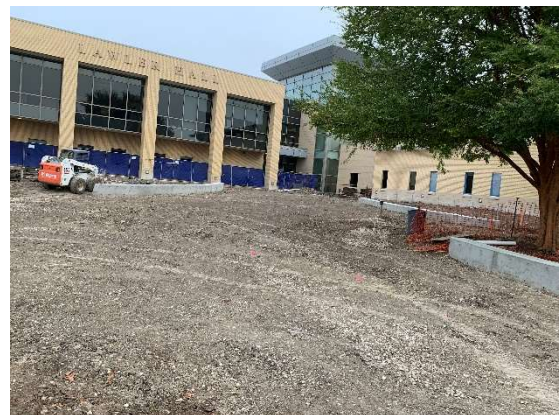
Prepping for Paving at Lawler Hall
