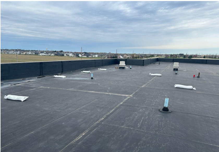
Sandbags holding it in place.
