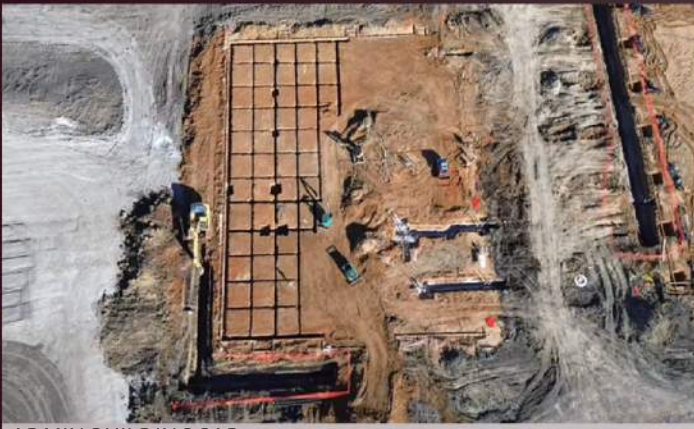
ADMIN BUILDING PAD
