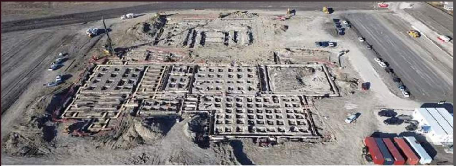
VIEW LOOKING NORTH
