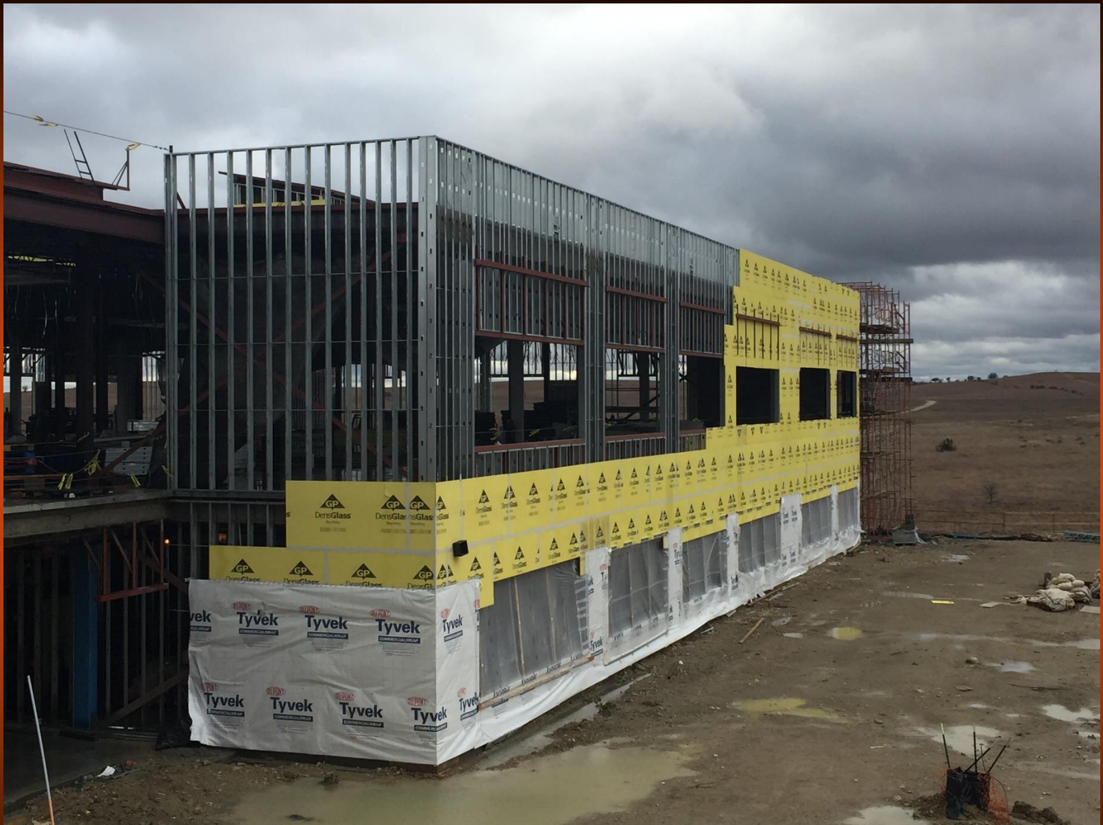
Elementary 5 Area A – Exterior Framing & Sheathing
