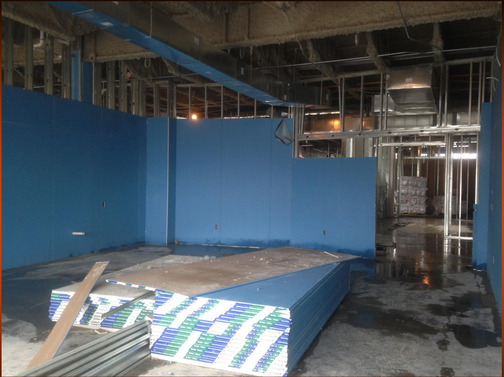
Elementary 5 Area A – Sheetrock Installation
