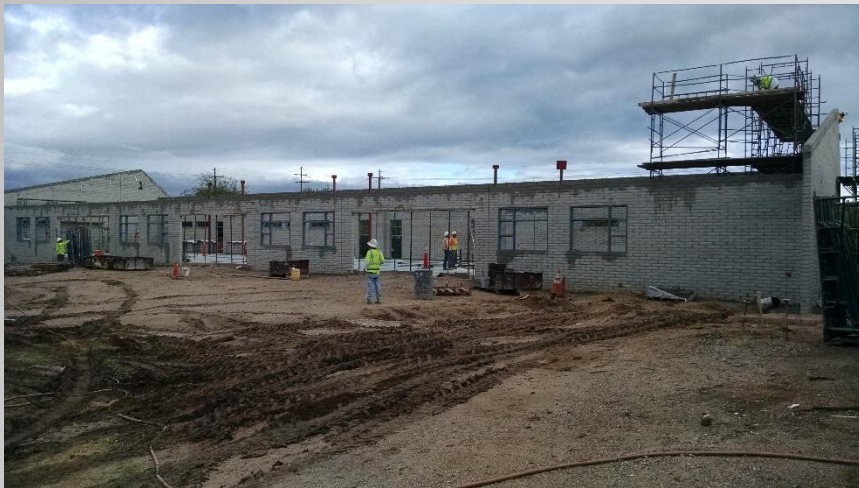
South Side Of New Building
