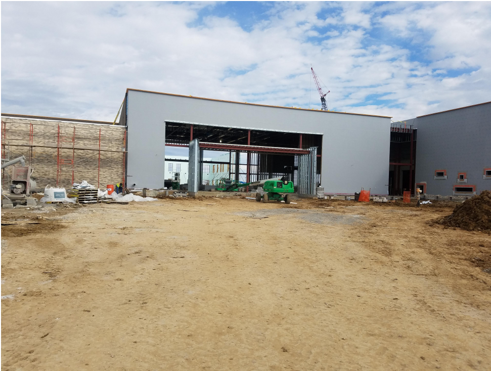
Cafeteria Plaza Entry.
