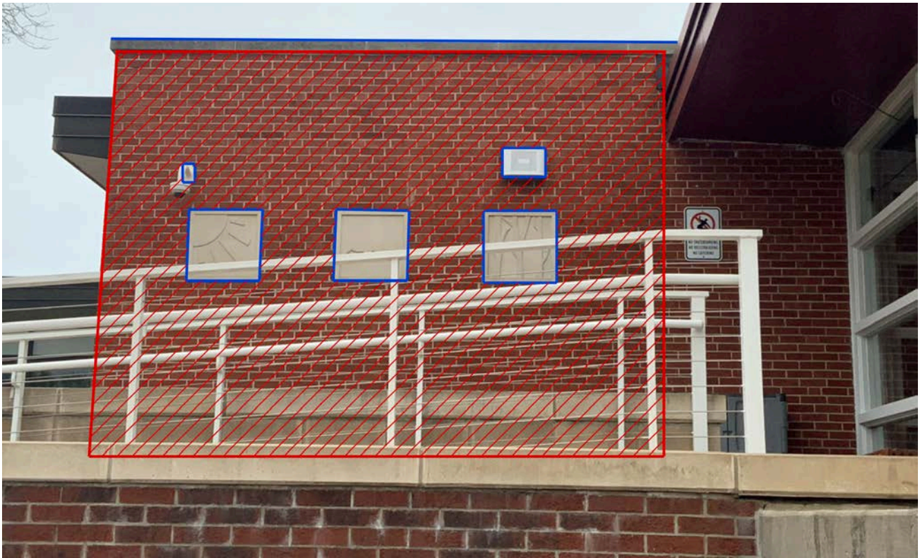
Note the deterioration of masonry directly below coping stones
