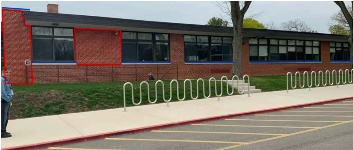
Note the deterioration of masonry directly below coping stones
