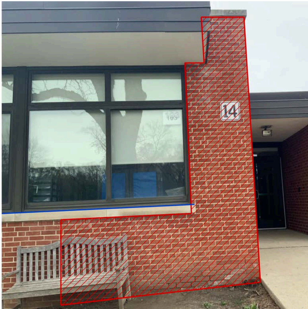
Note the deterioration of masonry directly below coping stones
