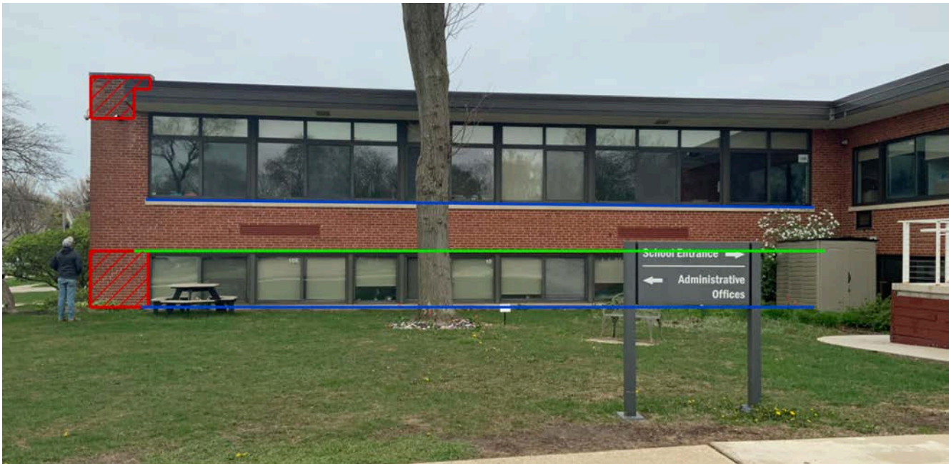
Note the deterioration of masonry directly below coping stones
