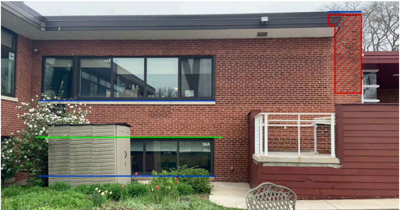
Note the deterioration of masonry directly below coping stones
