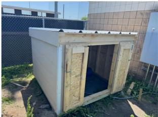
This little shed may not look like much, but it was constructed to protect a major irrigation pump in the district. The shed is outfitted with a heating system that will keep it from freezing up during the winter months.
